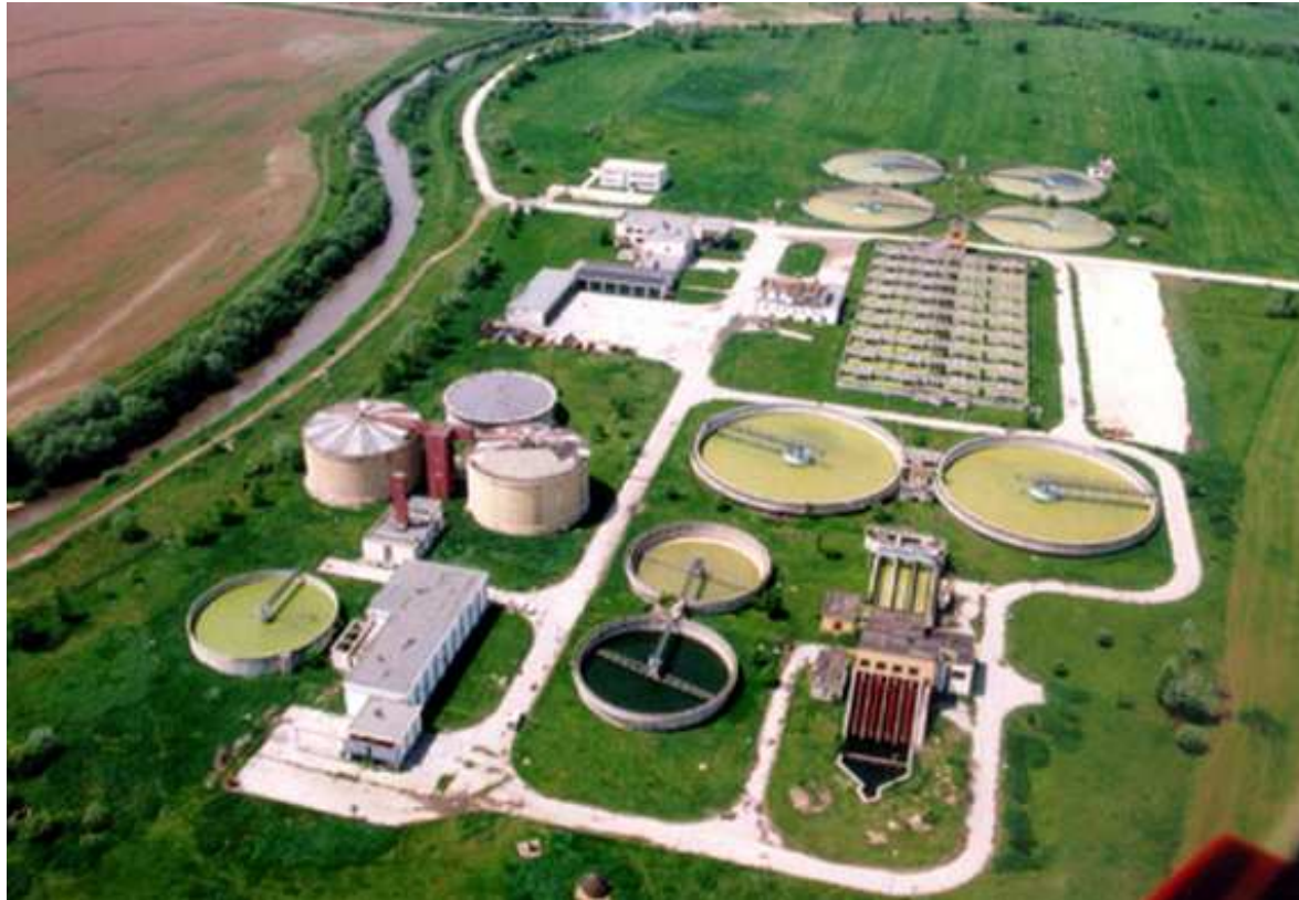
NATO's Sarajevo WWTP
